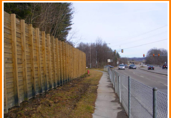
A temporary safety wall was built to prevent more rock from falling across the sidewalk and road.
