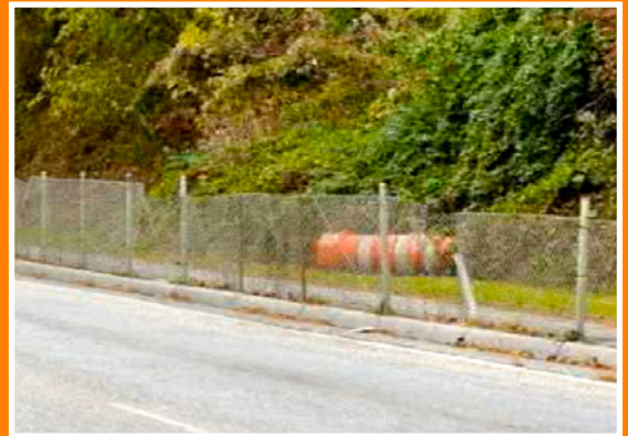
The chainlink fence that ran along the sidewalk's edge was damaged in places by vehicles, demonstrating its lack of protection for pedestrians on the sidewalk.
