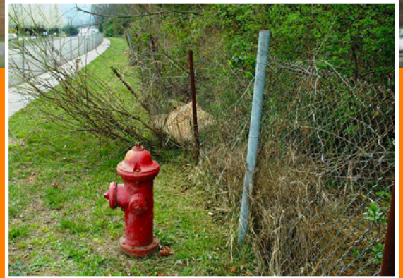
Falling rocks had become a life safety concern, with some rocks falling across the sidewalk and onto the roadway.
