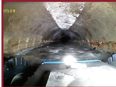
CCTV (Closed Circuit Television) INSPECTION
